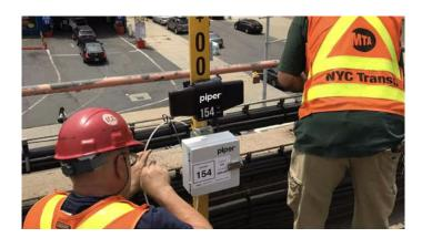
Piper team members were present in NYC and near the trackside during the installation process to address any questions and resolve issues promptly. Anchors were installed on the wayside of elevated tracks by attaching them to survey markers. In addition, anchors were attached to predetermined locations in tunnels using Piper's custom-developed bracketry.
